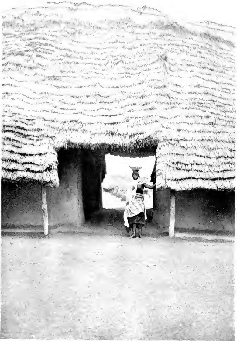
ENTRANCE TO THE "AFIN" OR RESIDENCE OF THE ALAFIN OF OYO, SHOWING TYPICAL YORUBA THATCHING.
